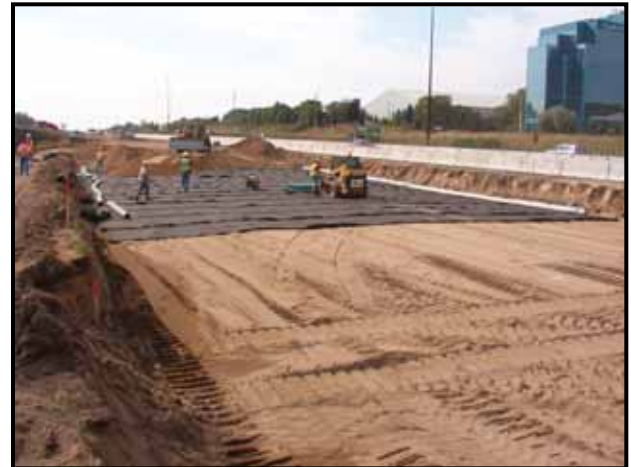
RoaDrain™ panels being deployed
