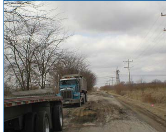
Bungalow Road had not been built to sustain the high volume of heavy truck traffic it has to support today.
