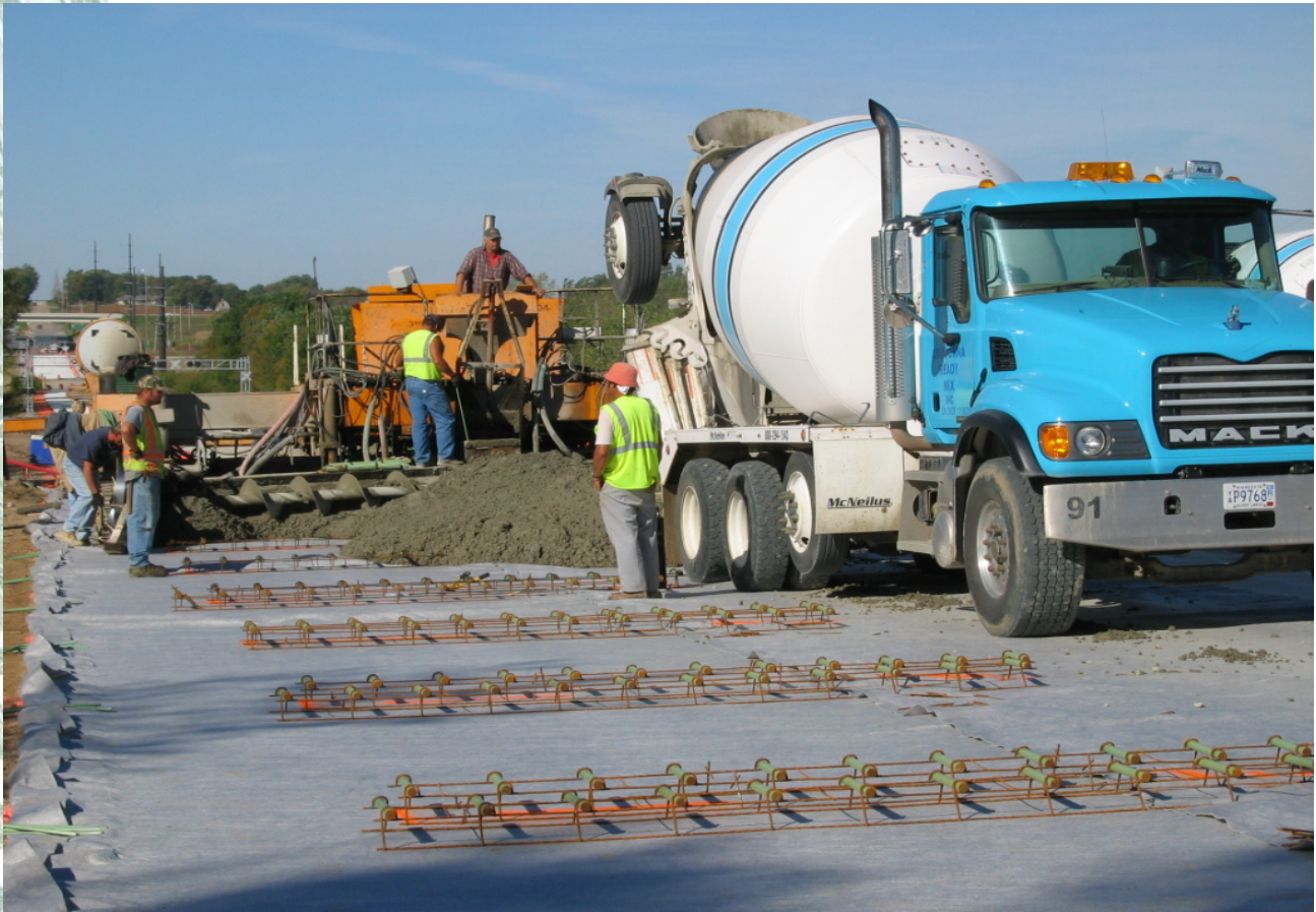
RoaDrain-T™ opens the door for flexibility to the paving process. The void-maintaining triplanar structure supports the weight of typical paving equipment without damage. This is not possible with conventional open graded based materials.
