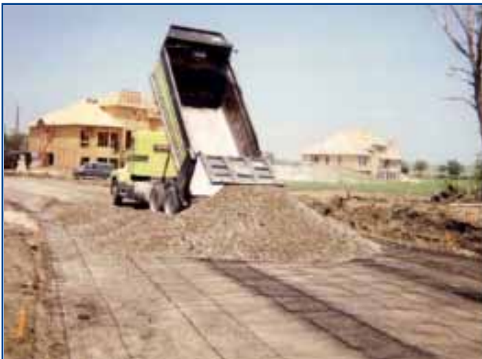
Photo 1: Back dump spread over geogrids
