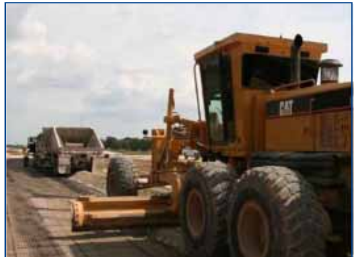
Photo 2: Bellydump spread over geogrids
